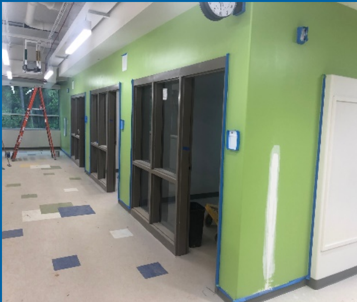
Gymnasium Drywall Final Patch and Paint
