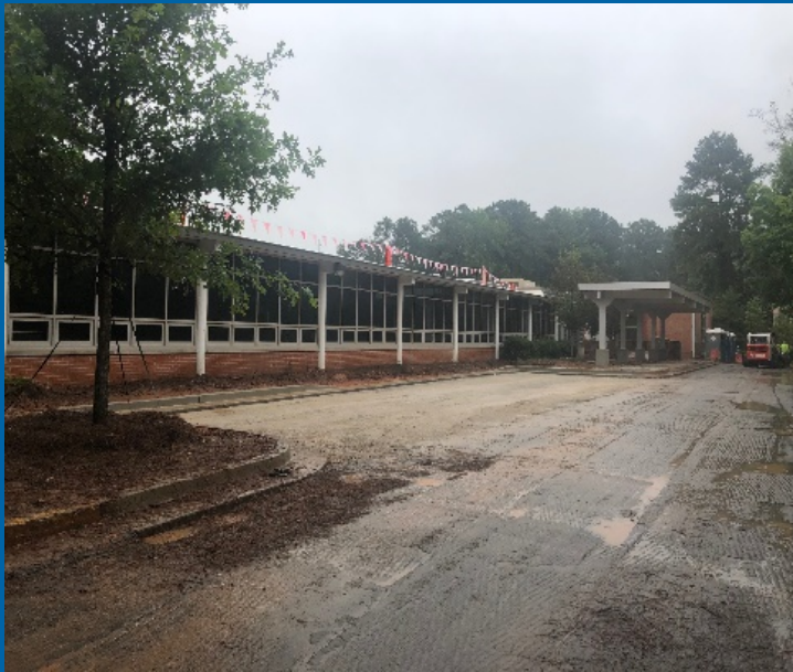
Handicap Parking Base and Curb Installed
